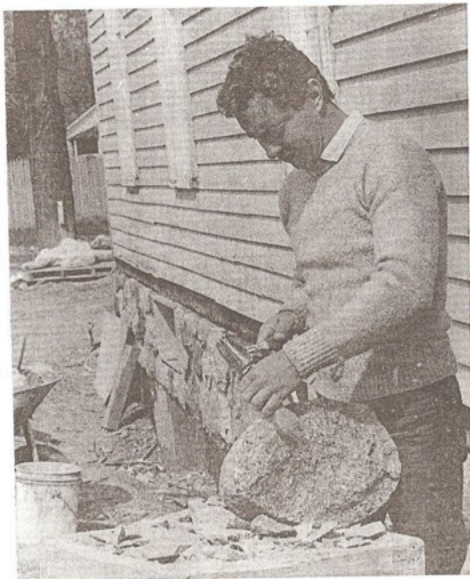
Trimming boulders into rough 5-inch squares for stone masonry is very physical work, but
