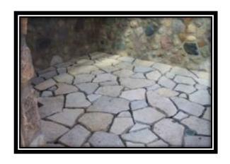
MUCH AS THE ORIGINAL STONE FROM THE FOUNDATION AS POSSIBLE. THIS REQUIRED US TO REMOVE ALL OF THE OLD MORTAR ATTACHED TO MOST OF THE STONE AND SPLIT EACH STONE SO THAT IT COULD BE RE-LAID ON NEW NARROWER FOOTINGS. THE PROJECT INCLUDED BLOCK WORK AND STONE FACINGS ON THE NEW OUTSIDE FOUNDATION WALLS, INSIDE
